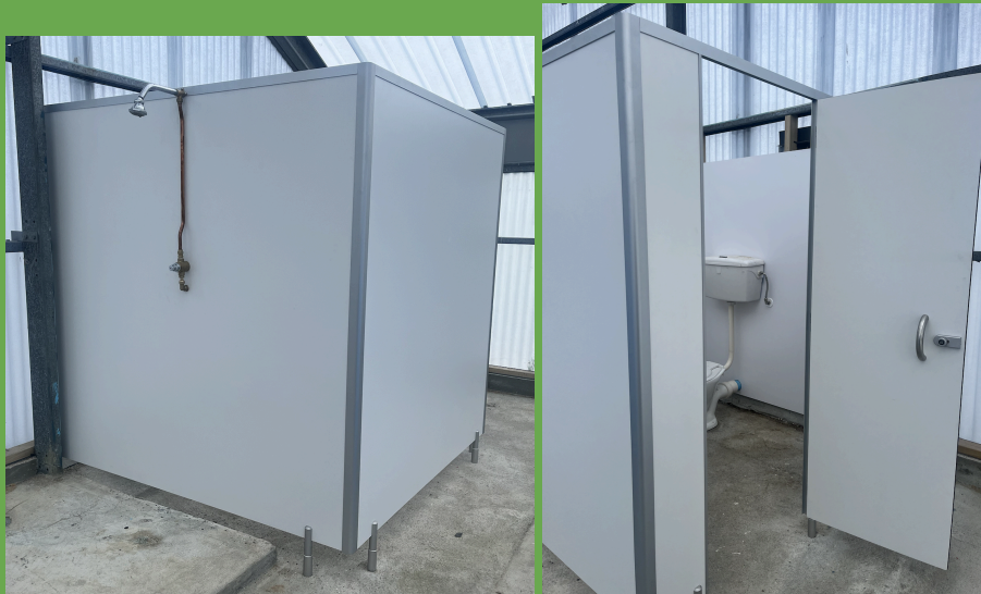
New toilet structure December 2024
